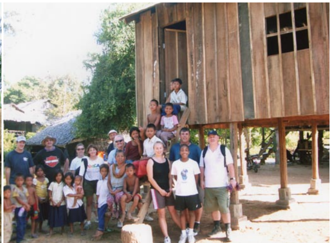
HOUSE BUILDING BY VOLUNTEERS
