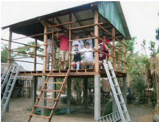
HOUSE BUILDING BY VOLUNTEERS
